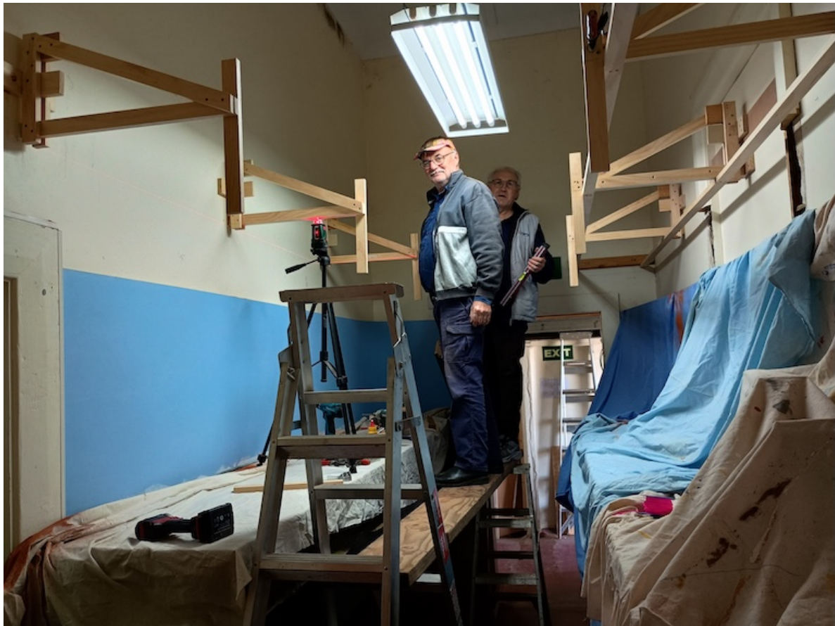
above: Wayne Hoskin and Danny Coppick standing on a plank while fixing the valance's framework in place on Saturday June 27. photo: A Mikolaj
